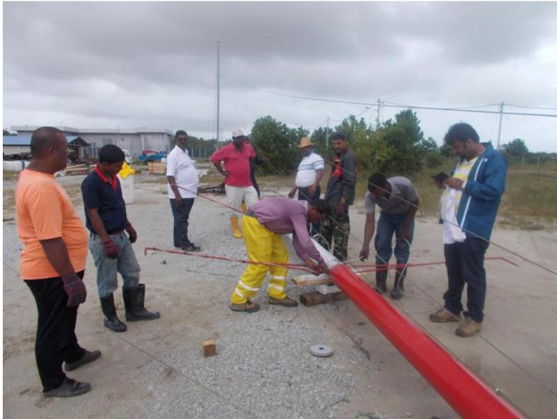
Tubular tilt-up Mast Assembly & Installation at Kelantan, Malaysia
